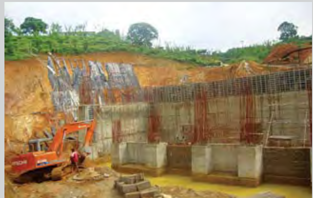
Power House (Under Construction)
