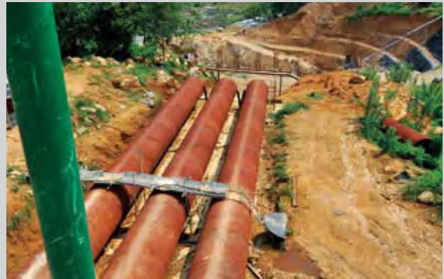
Penstock (Under Construction)
