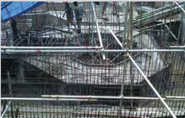
Power House (Under Construction)
