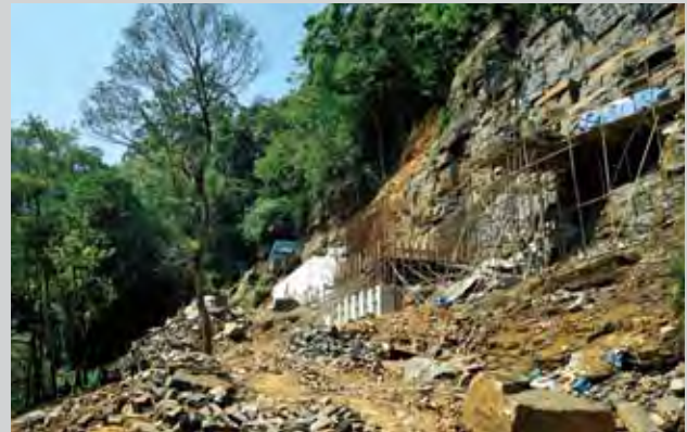
Forebay Tank (Under Construction)
