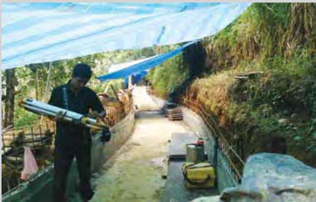
Head Race Channel (Under Construction)
