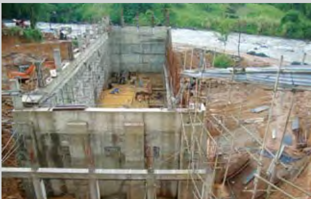
Power House (Under Construction)
