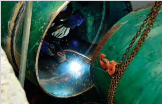
Penstock (Under Construction)
