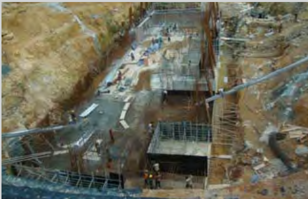
Power House (Under Construction)
