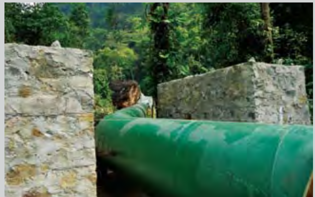
Penstock (Under Construction)
