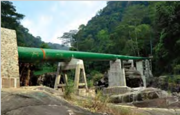
Penstock (Under Construction)
