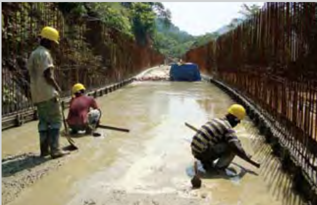
Head Race Channel (Under Construction)
