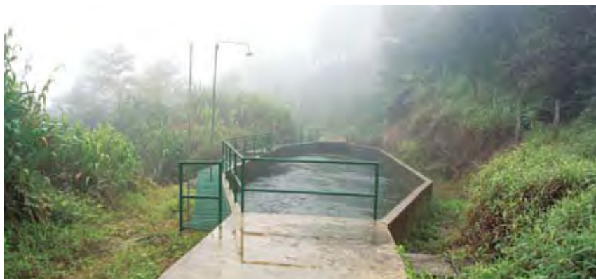
Erathna Project Sedimentation Tank
