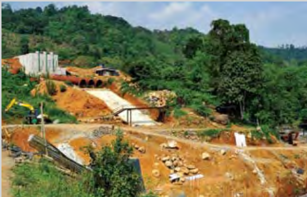
Forebay Tank (Under Construction)
