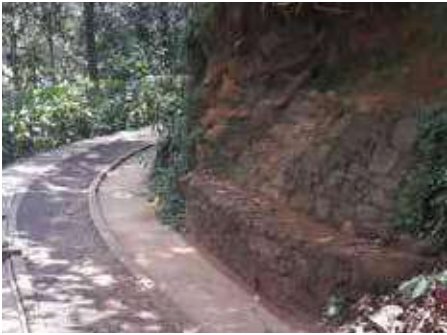
Retaining wall protection to avoid soil erosion
