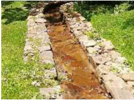
Spill water drainage system to avoid soil erosion
