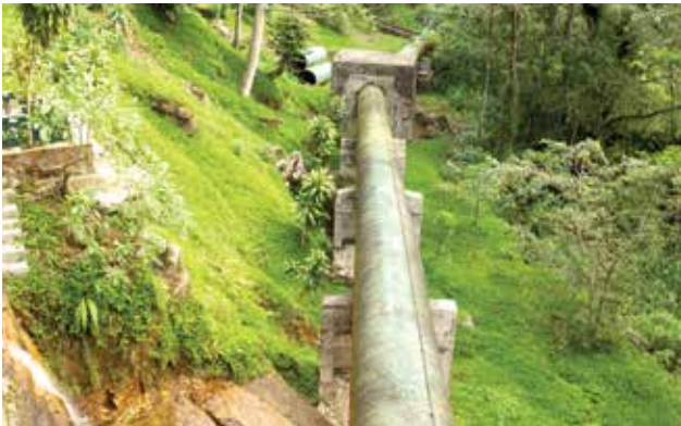
Efforts of surface vegetation developed to prevent soil erosion
