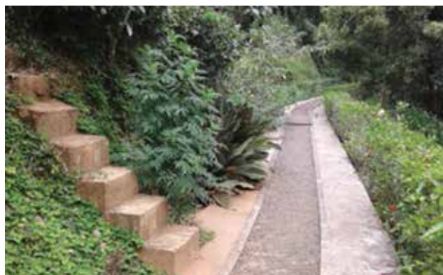
Concrete steps to facilitate movement of inhabitants across the channel
