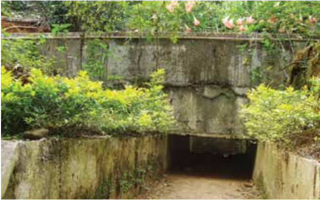
Drainage system constructed under the channel
