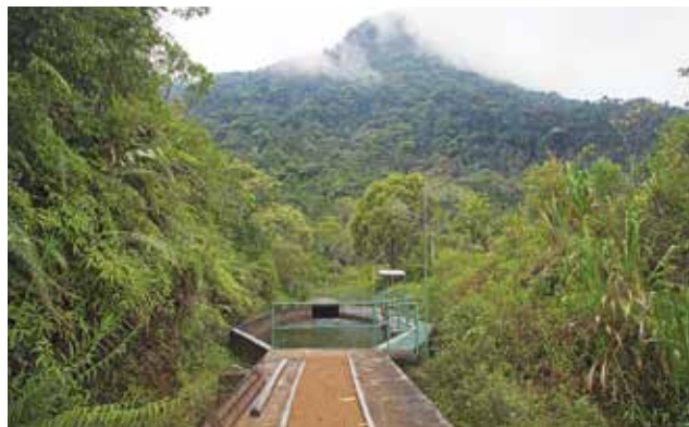
Closed head race channel and protective hand rails
