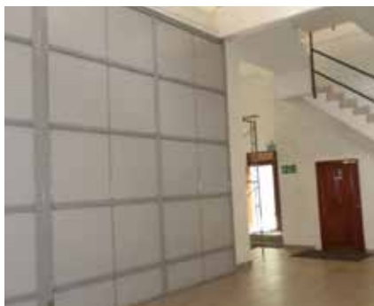
Noise Control Panel Installed at Erathna MHPP
