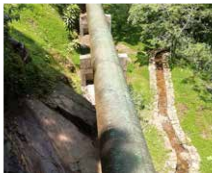
Surface vegetation and draining system to prevent soil erosion
