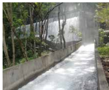
Concrete channel of Forbay spill to prevent soil erosion
