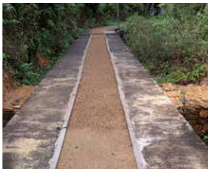
Closed channel and soil filled path to facilitate movement of inhabitants across the channel
