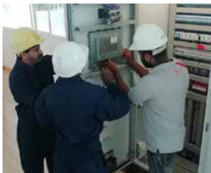
Replacement of touch panel at Kiriwaneliaya plant
