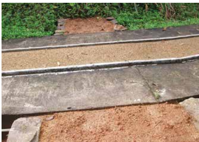
soil-filled path across channel for animal crossing
