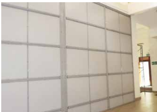
Noise Control Panel Installed at Erathna MHPP
