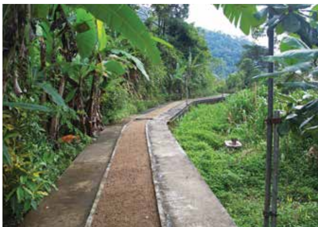
Head Race Channel closed with a concrete slab
