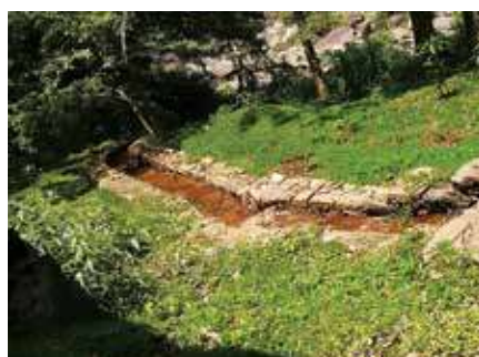
Surface vegetation and draining system to prevent soil erosion
