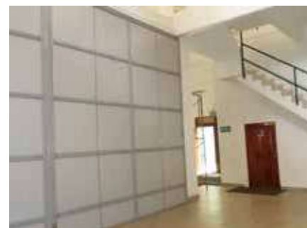
Noise Control Panel Installed at Erathna MHPP
