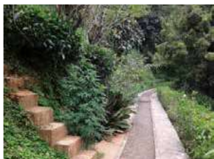
Concrete steps to facilitate movement of inhabitants across the channel
