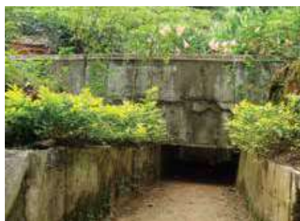
Drainage system constructed under the channel
