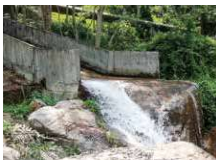
Concrete channel of Forbay spill to prevent soil erosion
